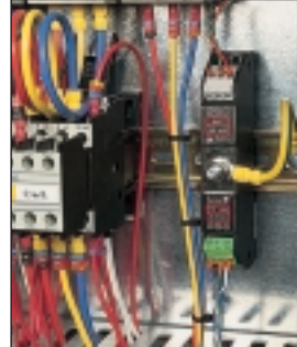
ESP 30E installed on top hat DIN rail inside a process control cabinet.
