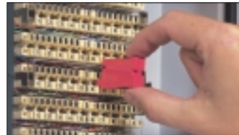
Having pushed the ESP KE10 earth bar on to the disconnection modules' earth points, firmly push an ESP KS06 (or ESP KS15, ESP KS30 or ESP KS50) into each line/pair requiring protection.
