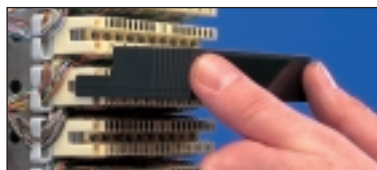
Firmly push an ESP K10T1 (or ESP K10T2) into each disconnection module requiring protection, so that it clips securely into the earth point, at each end of the module.
