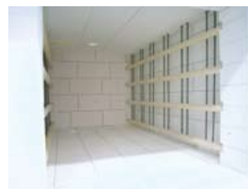
Protective screen in front of heating elements for protection against mechanical damage
