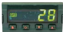
Over-temperature limit controller
