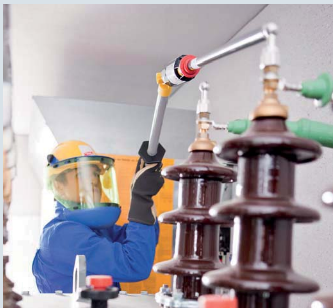
PHE III indicator with test prod, universal gear coupling and insulating stick
