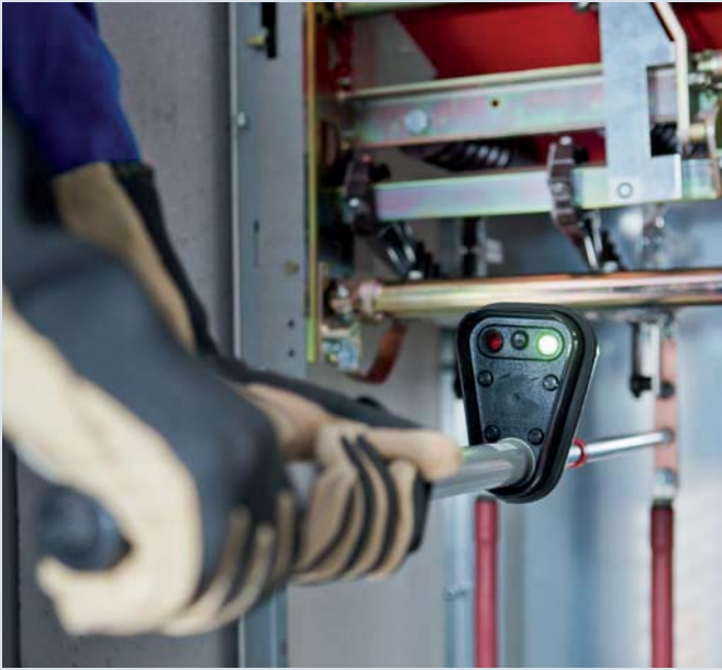
PHE voltage detector with visual indication
