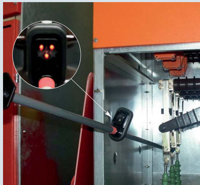
PHG II voltage detector used in a type-tested switchgear installation
