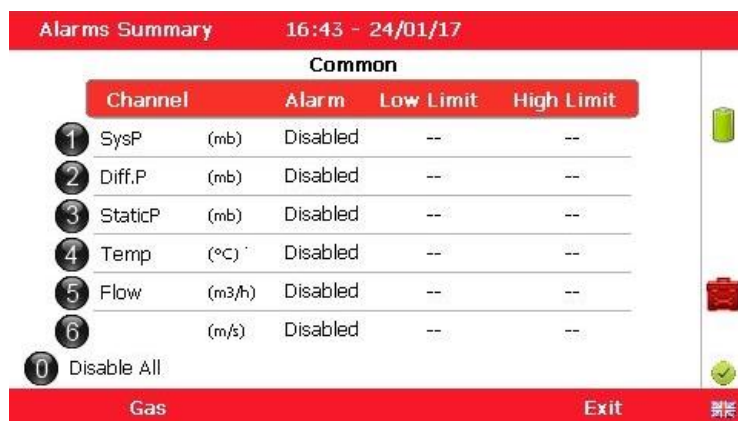
Set secondary alarms
