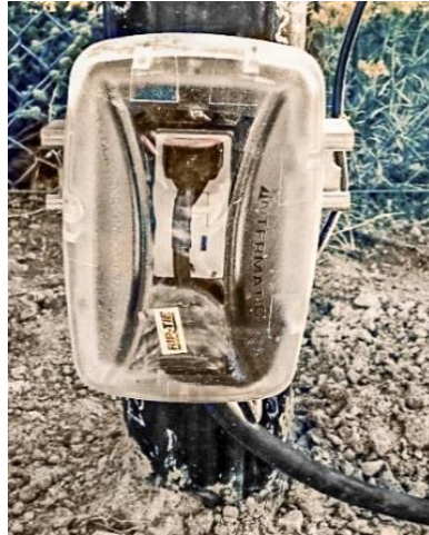
Figure 9: Water resistant/waterproof outdoor receptacle enclosure
